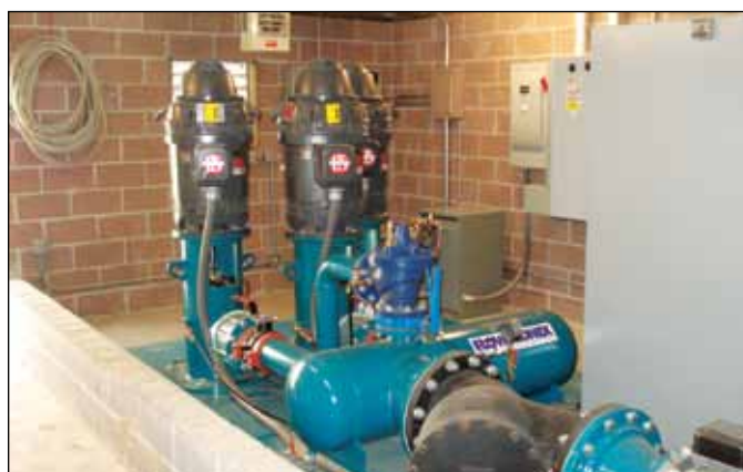
Figure 3-8. Vertical turbine pump station installation. Source: EC Design Group, LTD.
