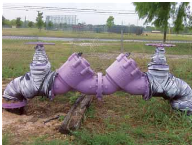
Figure 3-2. RPZ backflow prevention device. Source: EC Design Group, LTD.
