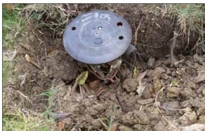
Figure 3-11. Poor sprinkler installation. The soil was not properly backfilled and compacted. Source: EC Design Group, LTD.
