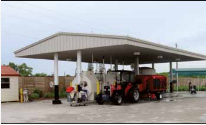
Figure 10-1. Covered fuel island and equipment washing area. Source: Terry Buchen.
