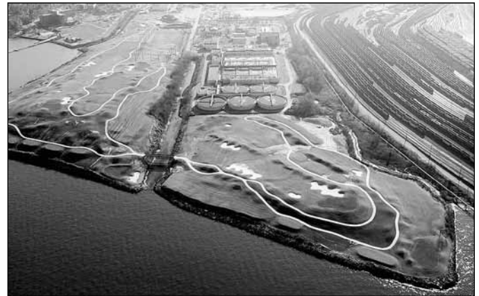
Figure B-5. Aerial view. Source: George Golf Design.
