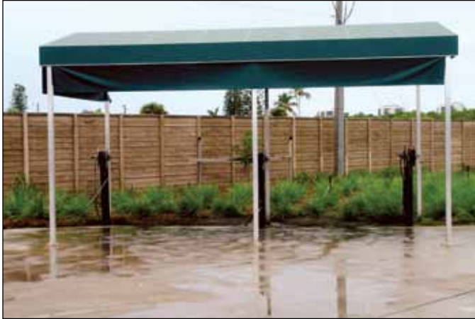
Figure 10-3. Equipment wash rack with air hose pre-cleaning area. Source: Terry Buchen.
